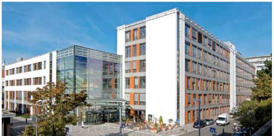
University Hospital Mainz Powder Coating with chrome-free Pre-treatment: PBS Schreiner GmbH & Co. KG / Germany
