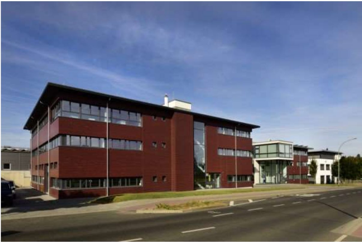
Headquarters of Clean-Lasersysteme GmbH in Herzogenrath
