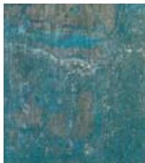
Steel surface with adhering tinder largely rust free
